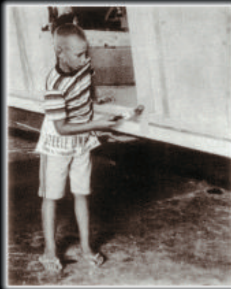
Johnnie Crean building a trailer in the 1950's.
