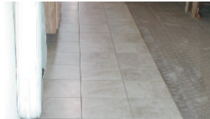
Ceramic Tile Flooring – more durable than linoleum, and looks more sophisticated as well.
